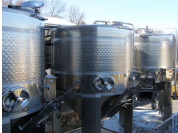
External Stainless Steel Tanks
